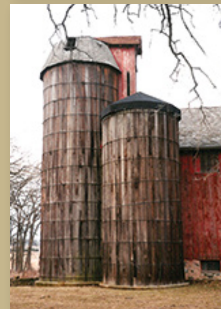
Peterson Farm, 4112 McCullom Lake Road, McHenry. Landmarks Illinois awarded a Preservation Heritage Grant in 2006 to restore the silos and repair the main barn.
