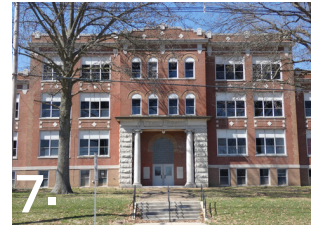
7. Former Collinsville Township High School Collinsville
