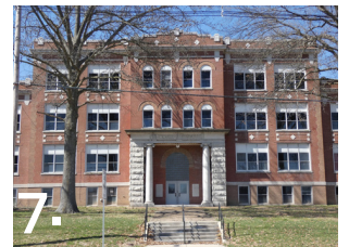
7. Former Collinsville Township High School Collinsville
