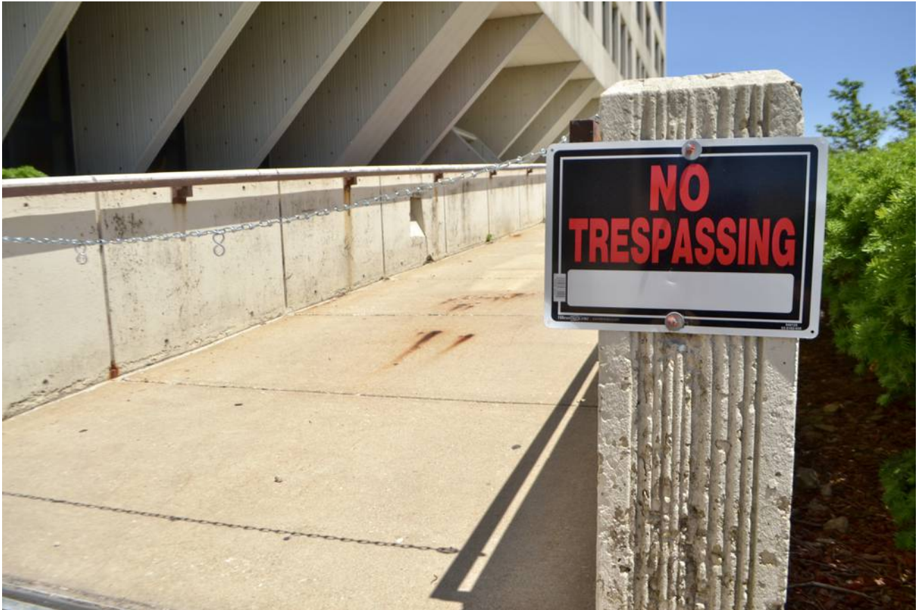
The old Will County Courthouse sits vacant in downtown Joliet on June 7, 2022. (Alex Ortiz)
