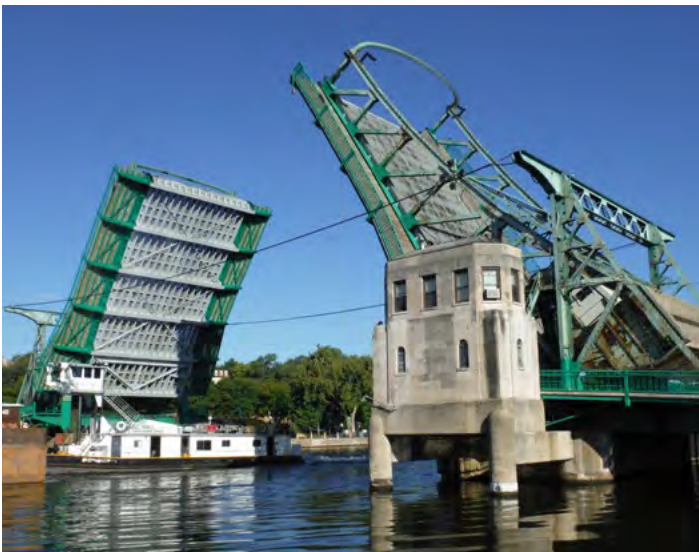
Jefferson Street Scherzer Rolling Lift Bridge, Joliet, IL
