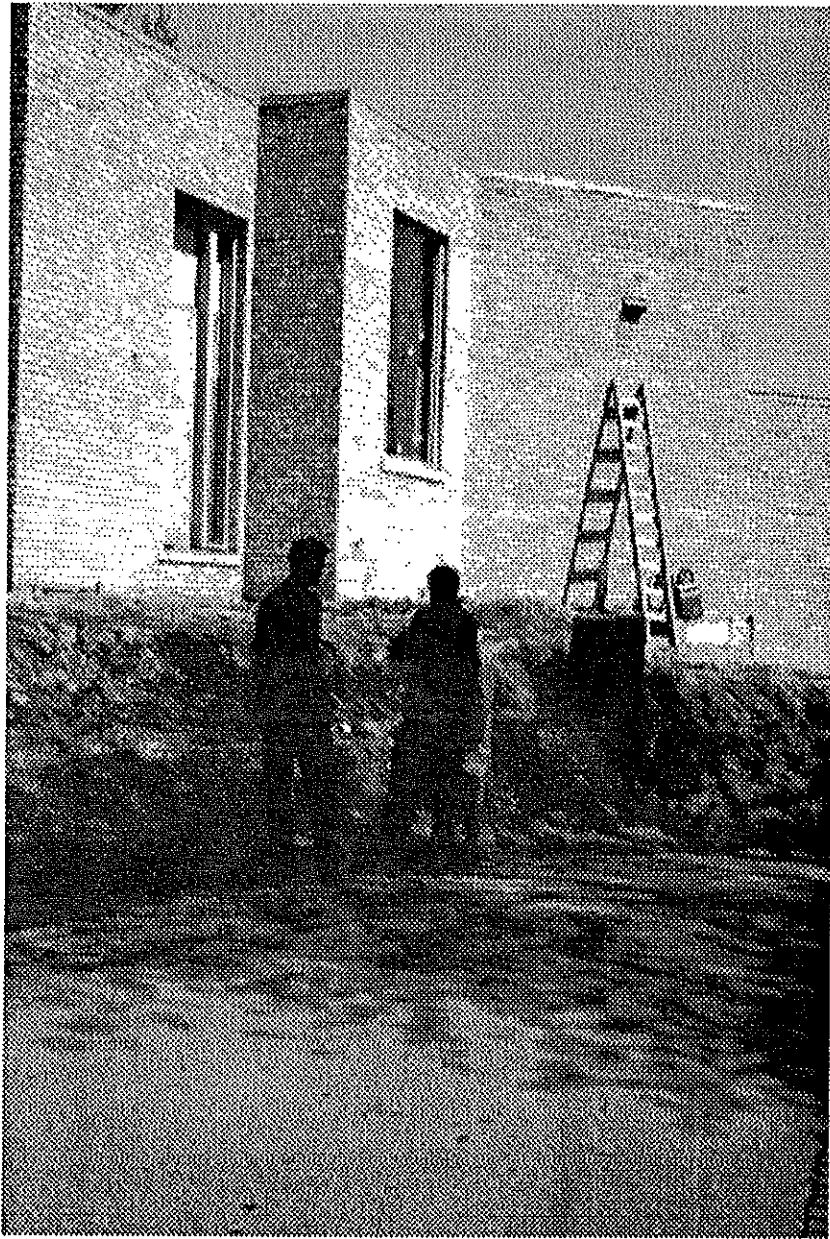
Figure 4. Kuh discusses design of retaining wall with architect and landscape contractor, 1958
