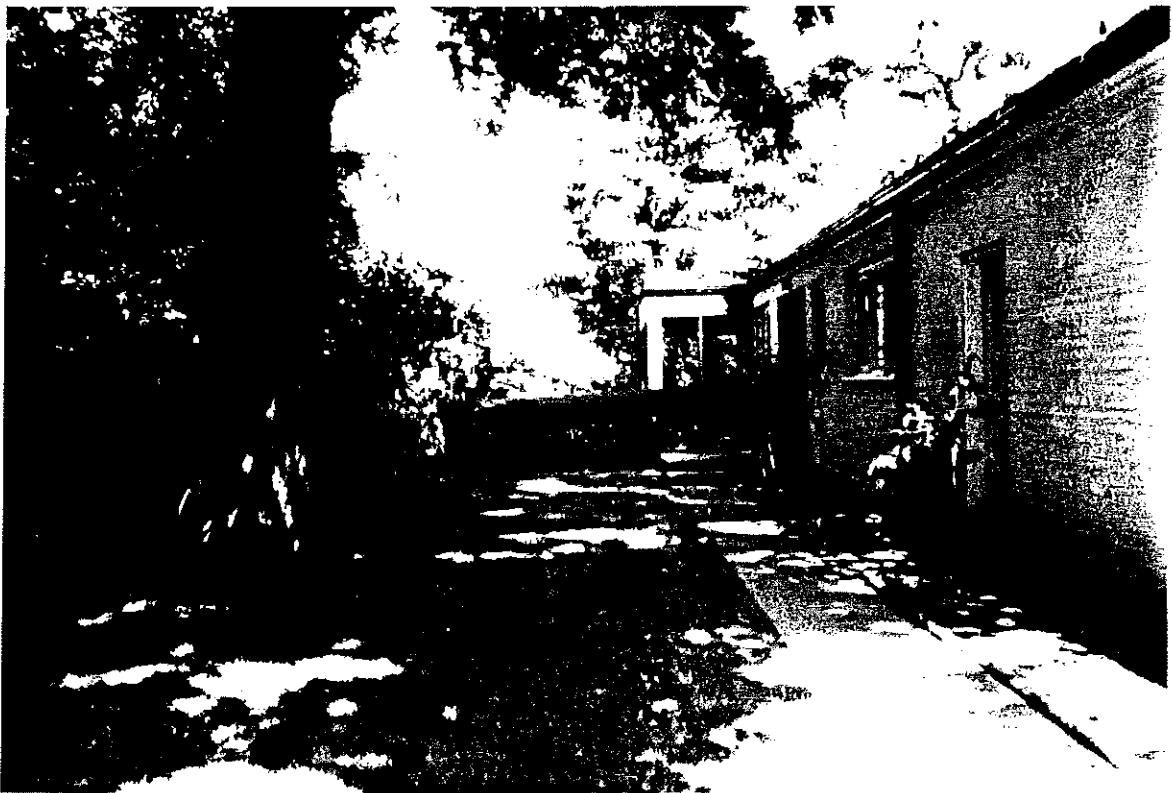
Figure 16. Service Area path connecting to the kitchen entrance.
