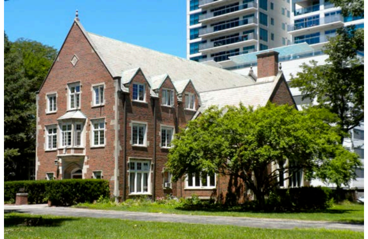
The former Alpha Delta Phi house was demolished.
