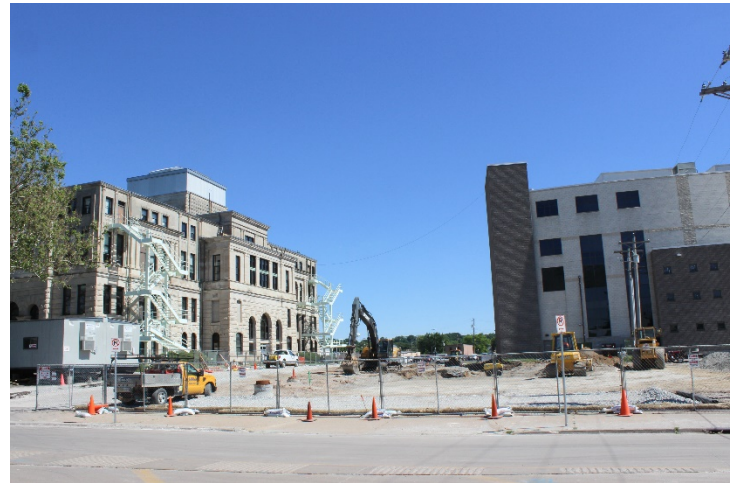
The new annex under construction with the historic courthouse (left) next door. Credit: Landmarks Illinois
