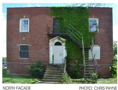
Based on visual inspection, the consulting team for this report felt that despite the building's deteriorated appearance, the basic structure is sound and in need of what appears to be only minor repairs due to the sturdy concrete construction. A new roof with masonry repairs and tuckpointing will provide decades of service to the new users.
