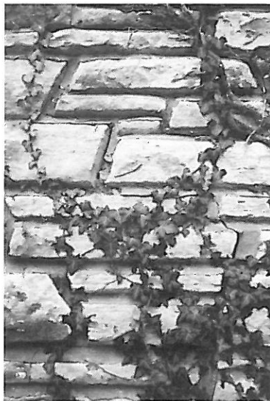
Certain types of ivy project needle-like probes into mortar joints and masonry. Growth of such ivy accelerates deterioration of the stone wall. Photo by Harry Hunderman, AIA.
