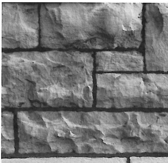
A detail of the tower wall at St. James Cathedral before restoration clearly shows the inappropriate repointing which had taken place in the past. The original joints were generally less than 1/8 inch wide, but repointing with a very dark mortar overran the joints by a large margin. Wiss, Janney, Elstner Associates, Inc. photograph.
