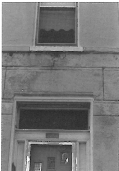
Deterioration is evident in the stone panels below a window sill course on this rowhouse. The window sill itself has been replaced, and the adjacent sill course shows spalling. Water collecting and passing through open joints in the sill to the stone panels below is likely the principal cause of deterioration. Wiss, Janney, Elstner Associates, Inc. photograph.
