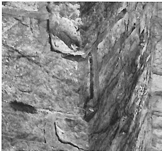
The limestone butresses at Christ Church in Winnetka have been damaged by the effects of freeze-thaw cycling. Pressure from the expansion of freezing water within the wall has caused the mortar joints to open up and step cracking to occur throughout the stonework. Photo by Harry Hunderman, AIA.
