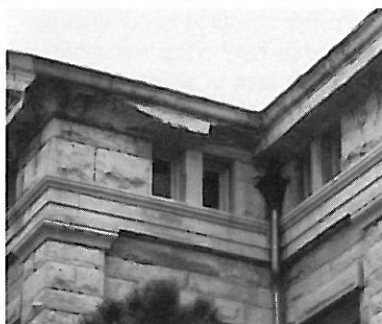
Cornice and upper wall at Rock Island Arsenal. Results of testing on treated samples indicated that conservation treatments significantly improve water absorption and compressive strength of the dolomite limestone. All photos courtesy ProSoCo, Inc.
