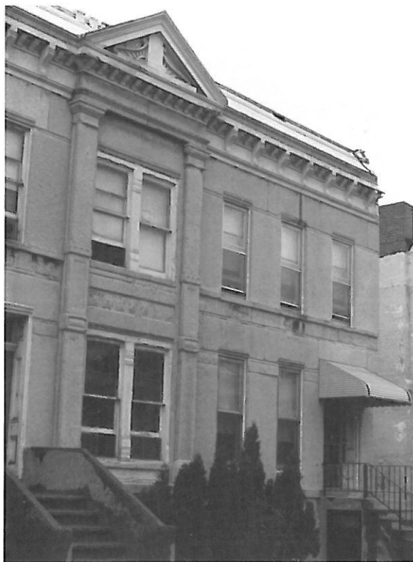
Row houses on West Bowler Street in Chicago's Tri-Taylor Historic District were constructed in the 1870s with Joliet-Lemont limestone panels attached to a brick wall. The cornice is ornamental sheet metal. The present condition of the limestone varies from house to house and sometimes from block to block. Wiss, Janney, Elstner Associates, Inc. photograph.
