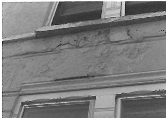
This rowhouse facade exhibits deterioration in an area of stone which has been painted. Improper use of coatings may contribute to the deterioration of limestone, since many paints are not vapor-permeable. Moisture is trapped within the stone substrate, contributing to damage from cyclic freezing and thawing. Common symptoms of this problem include peeling of the paint coating and spalling of the limestone. Wiss, Janney, Elstner Associates, Inc. photo.
