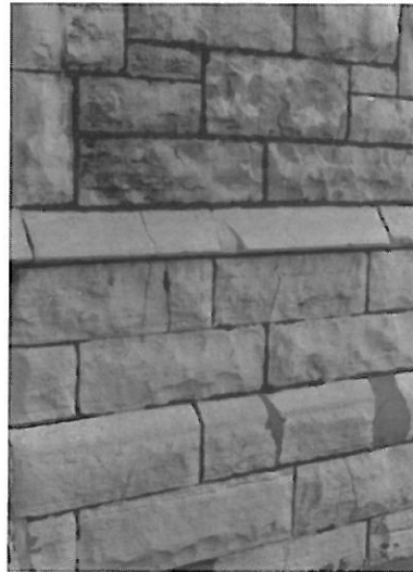
A detail of the tower at St. James Cathedral shows variation in color and texture of rusticated limestone blocks and the smoother sill course. Note localized cracking and old patches on this part of the wall. Much of the limestone was found to be in good condition, but open head joints and open joints along the top of the stone belt courses had led to water penetration and spalling of adjacent stone.
