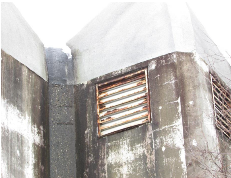
Figure 12. View of ridge between portal, as well as painted steel louver in wall
