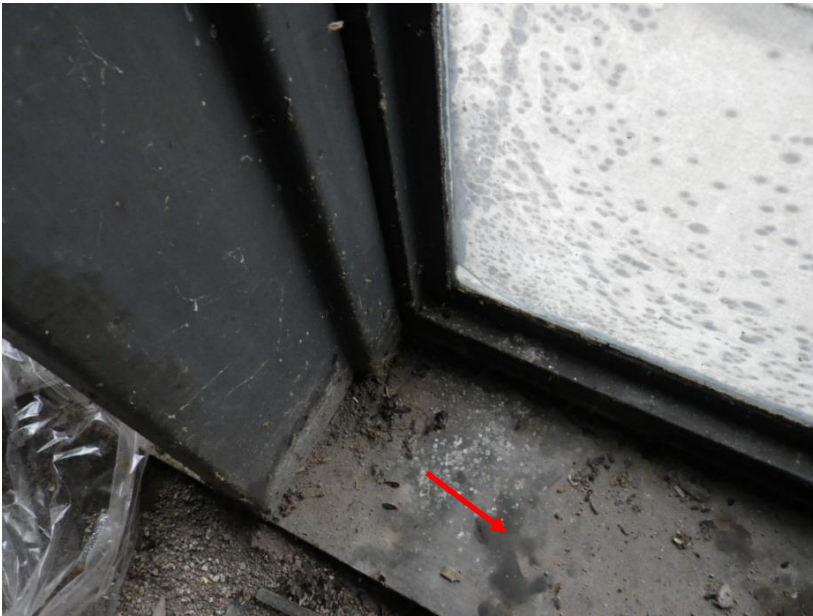
Figure 22. Water stains on bottom plate of curtain wall
