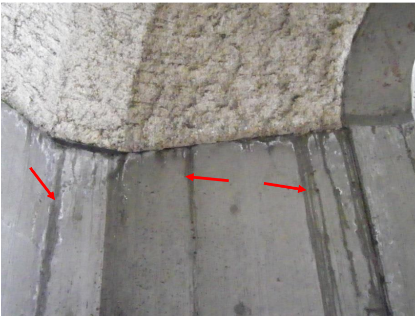
Figure 20. Indications of water leakage at transition between wall and ceiling area on interior
