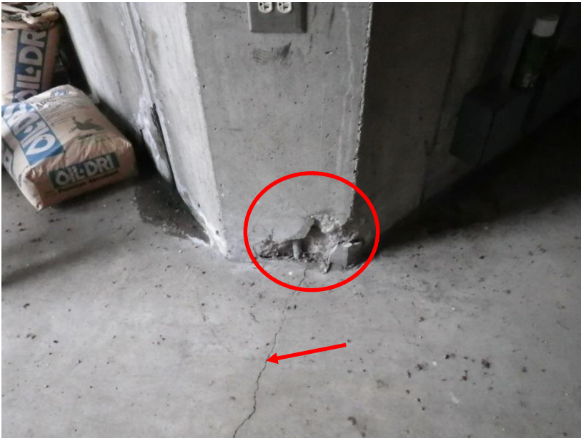
Figure 16. Spall at concrete at base of wall and crack in slab-on-ground
