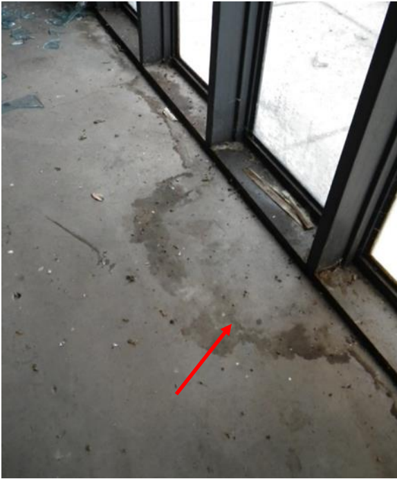
Figure 23. Indications of water infiltration and/or condensation on the slab adjacent to the curtain wall
