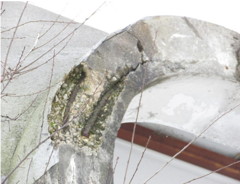
Figure 14. Spalled concrete at edge of end portal
