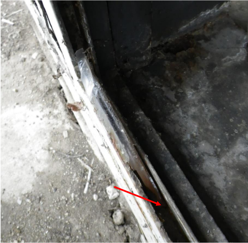
Figure 19. View of glazing pocket at broken lite in curtain wall at base. Note: no corrosion scaling is evident in the glazing pocket.
