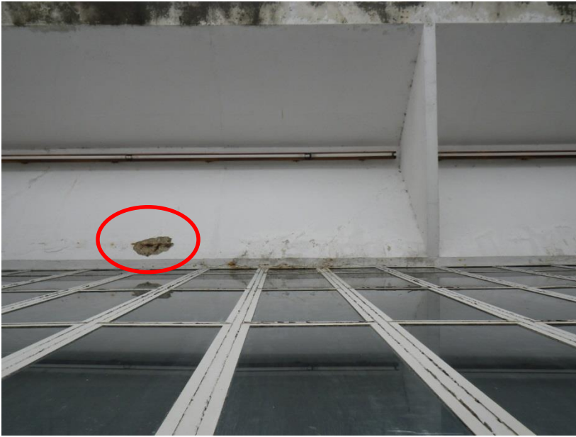
Figure 15. Spall in underside of overhanging portion of end portal on west facade
