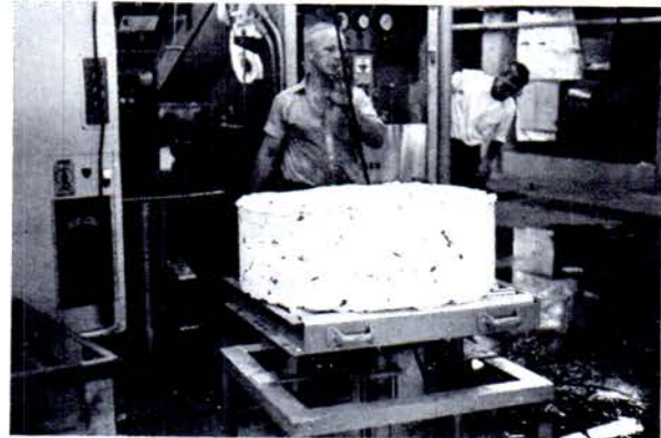
It might look like a birthday cake but it's really a tub full of wet wash that has been compressed in a special machine until all of the water is squeezed out. This "cake" is moved hydraulically since it is much too heavy for handling by hand. It is pushed into dryers that looked as if they were large enough to park a Volkswagen in. William Schwartz, now Acting Laundry Manager, operates the hydraulic controls. (ESH Photo)
