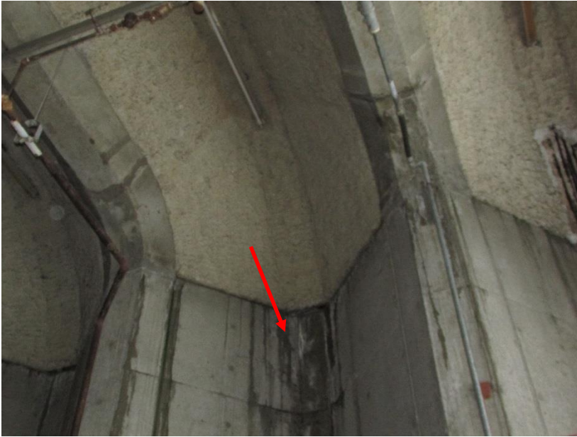
Figure 21. Indications of water leakage at transition between wall and ceiling area on interior
