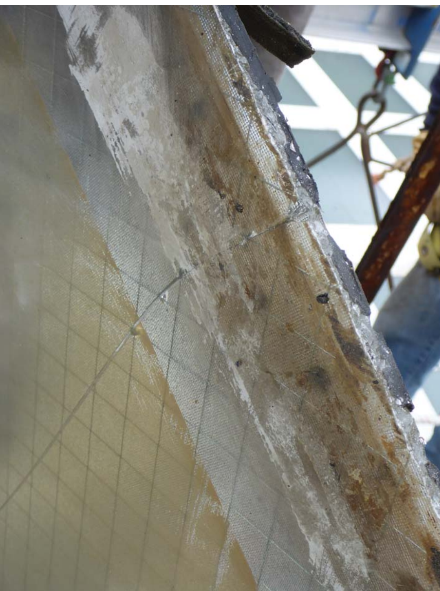
BROKEN WIRE GLASS
