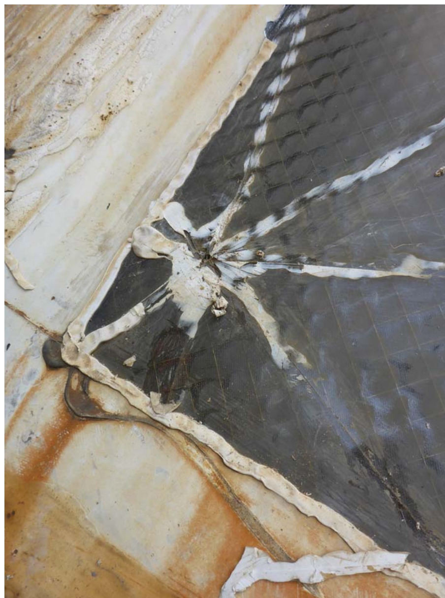
EXISTING WIRE GLASS WITH IMPACT DAMAGE
