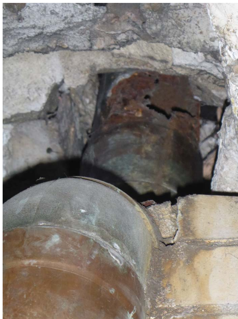
GALVANIZED DRAIN PIPE DETERIORATION DUE TO GALVANIC CORROSION
