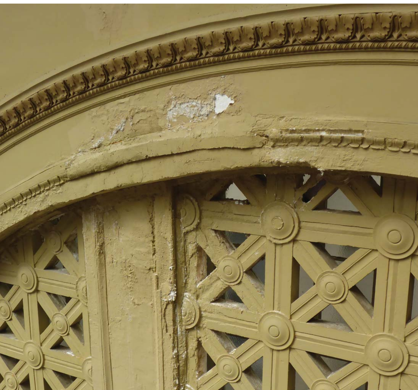
PLASTER DETERIORATION DETAIL AT NORTHWEST CORNER
