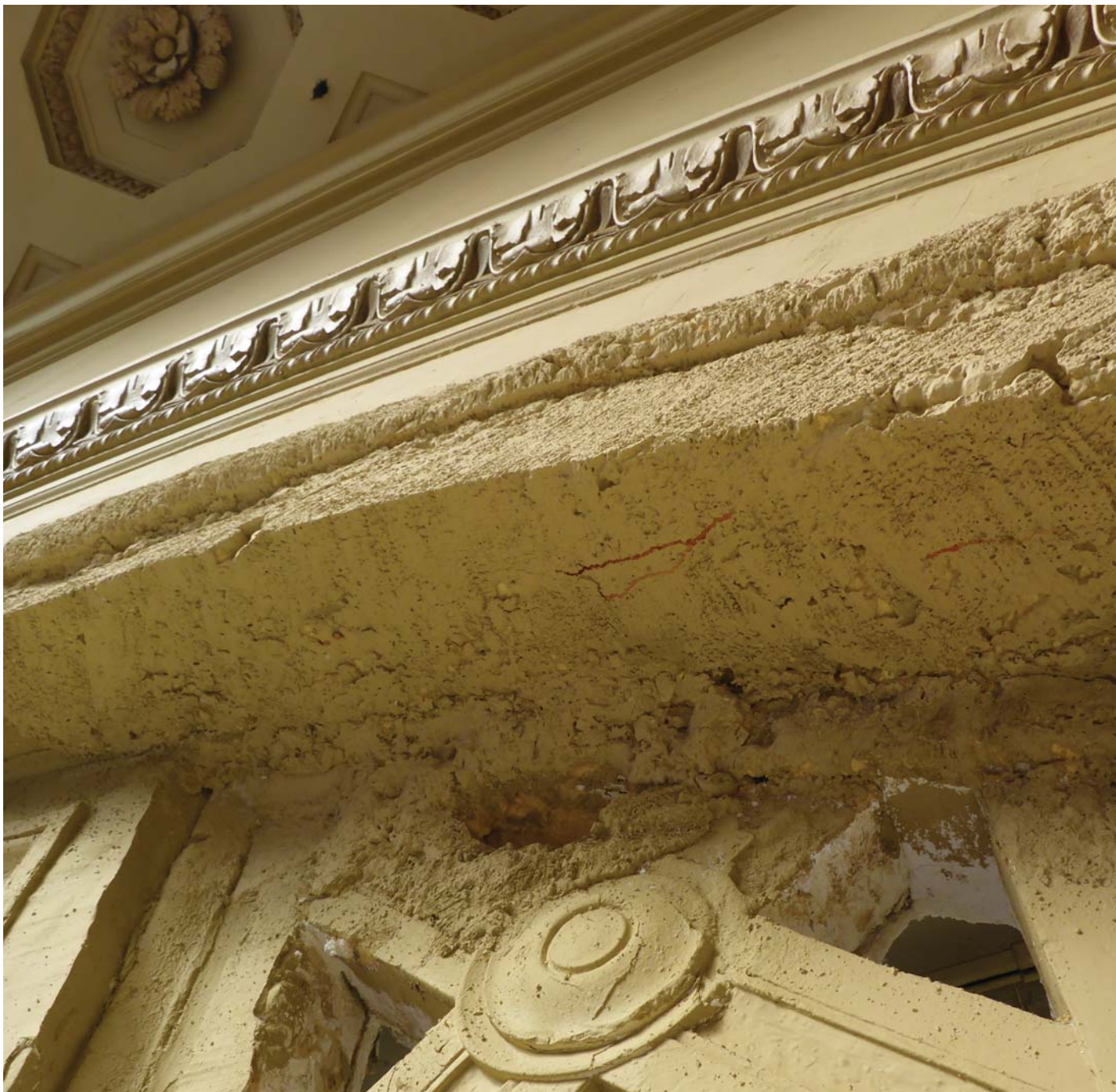
PLASTER DETERIORATION DETAIL AT NORTHWEST CORNER
