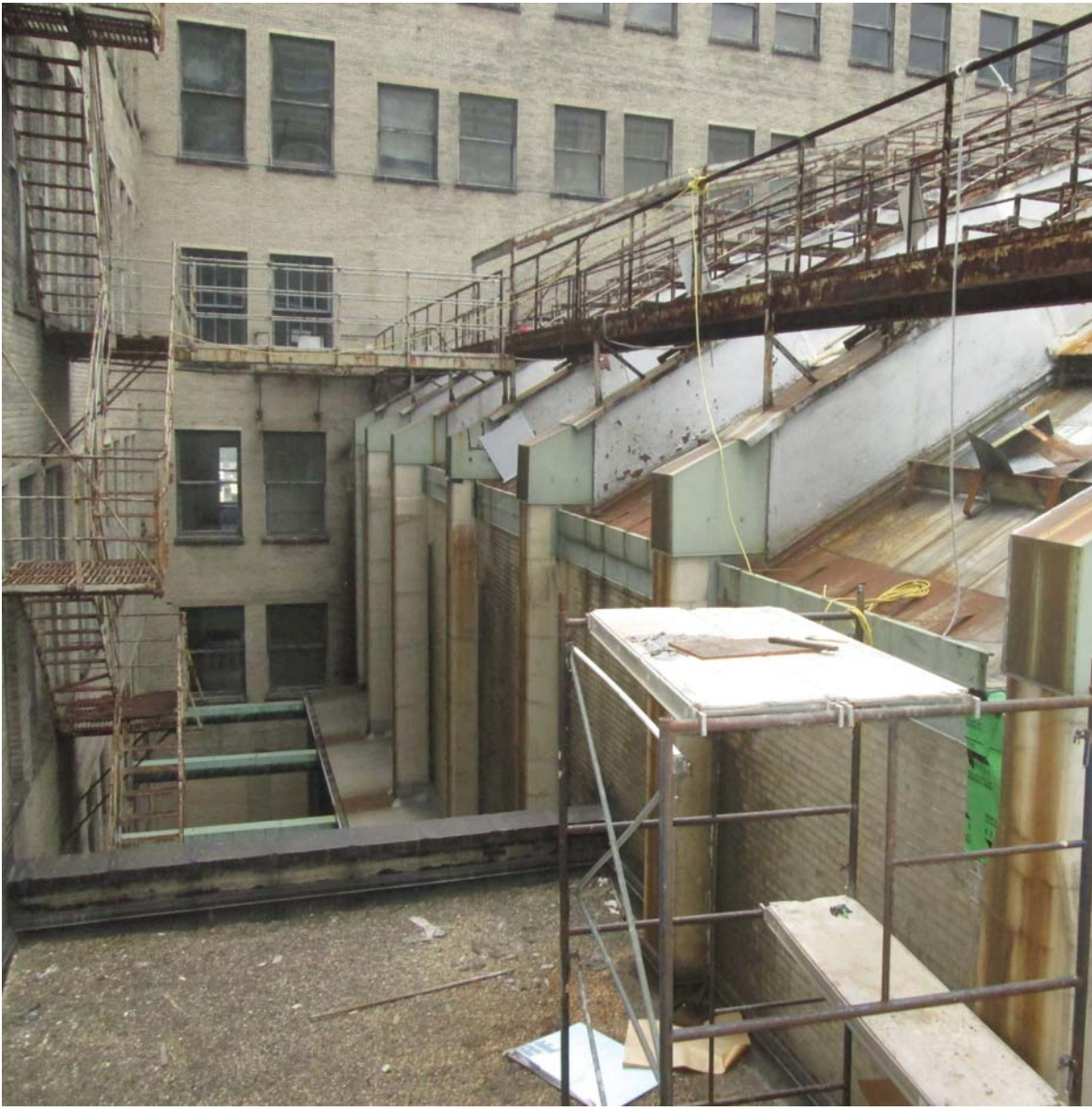
LIGHT COURT EAST SIDE
