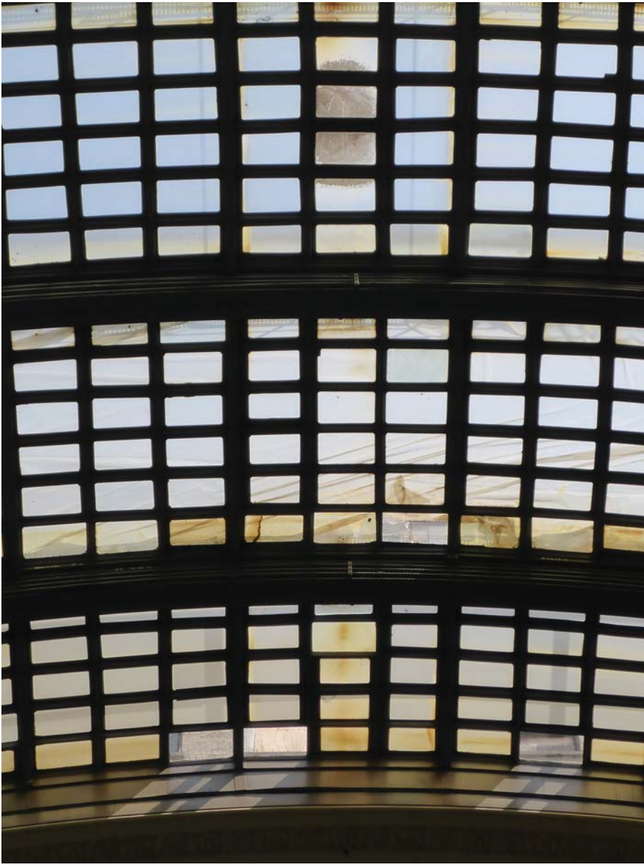
EXISTING SKYLIGHT FROM BELOW SHOWING EFFECTS OF WATER PONDING AND ADDED FLASHING BANDS
