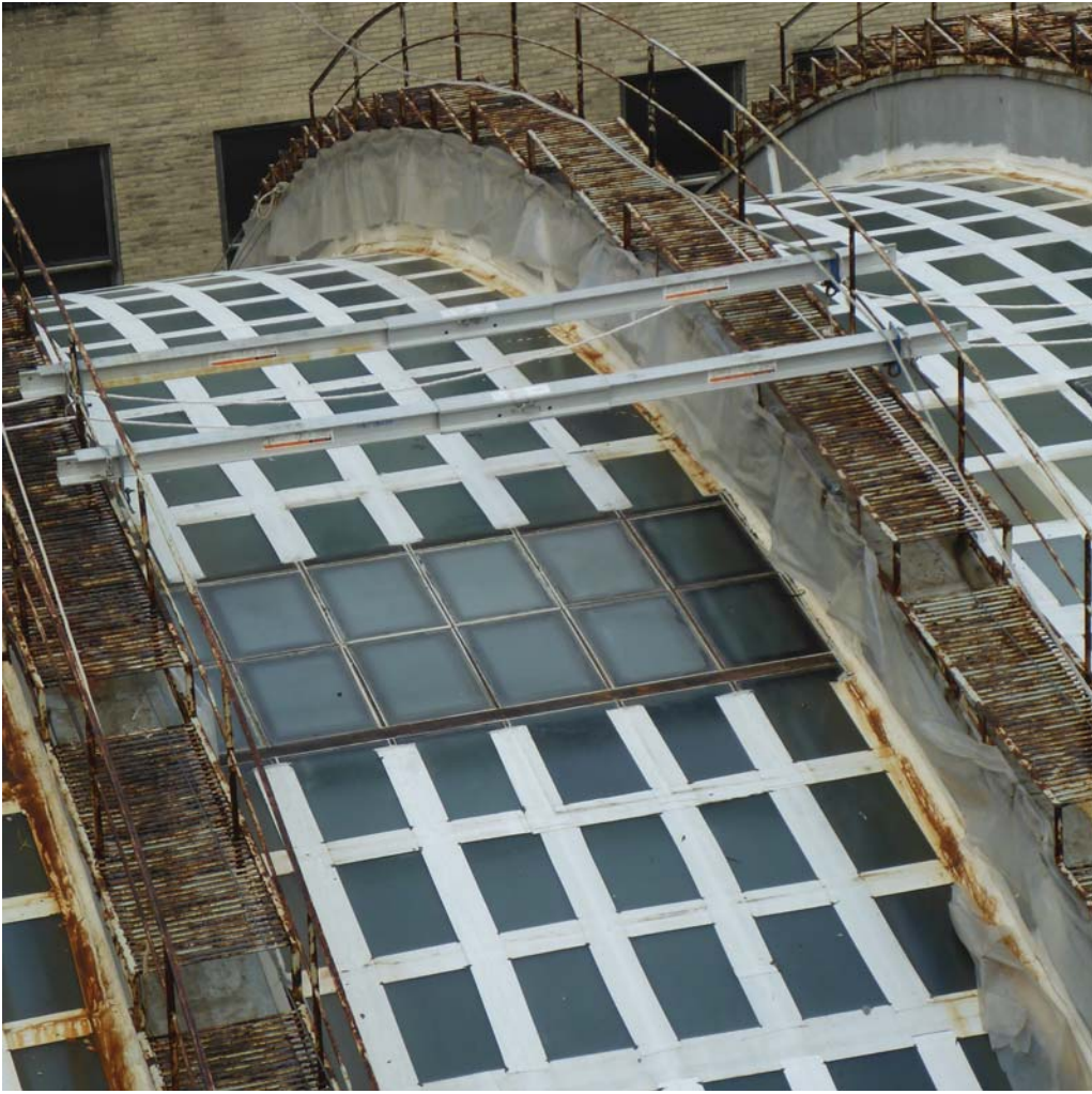
SKYLIGHT FROM ABOVE WITH SECTION OF OVERLAY FLASHINGS REMOVED
