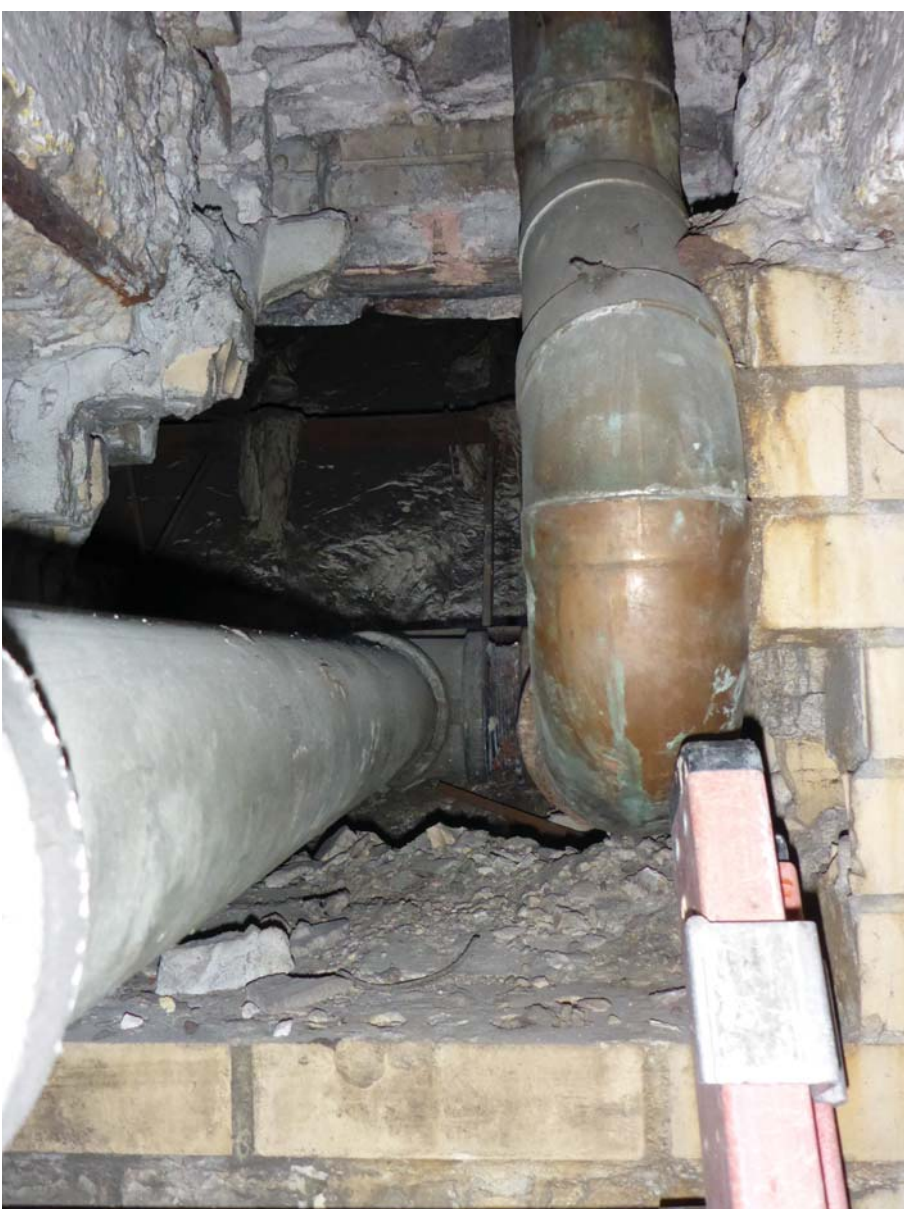
ORIGINAL CAST IRON DRAIN PIPE WITH TRAP AND VENT - SECTIONS REPLACED WITH COPPER AND GALVANIZED PIPE OVER TIME
