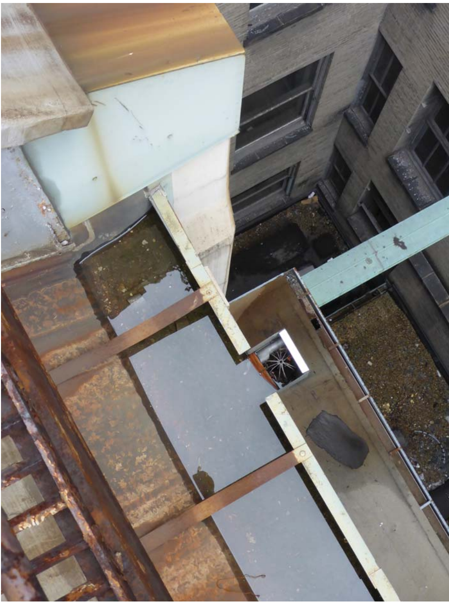
EAST GUTTER - STANDING WATER WHERE ORIGINAL DRAIN FAILED AND EXTERNAL DOWNSPOUT WAS ADDED
