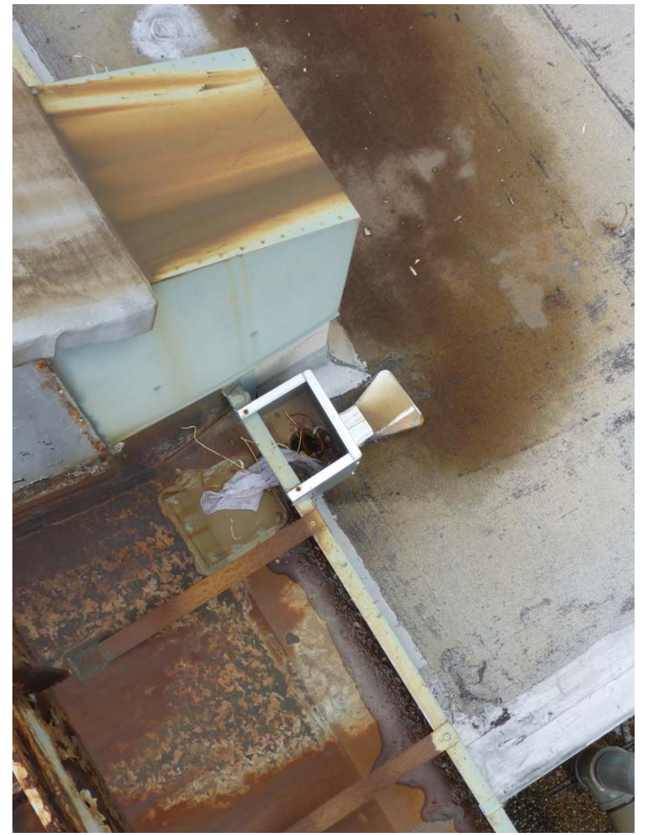
EAST GUTTER - STANDING WATER WHERE ORIGINAL DRAIN FAILED AND EXTERNAL DOWNSPOUT WAS ADDED
