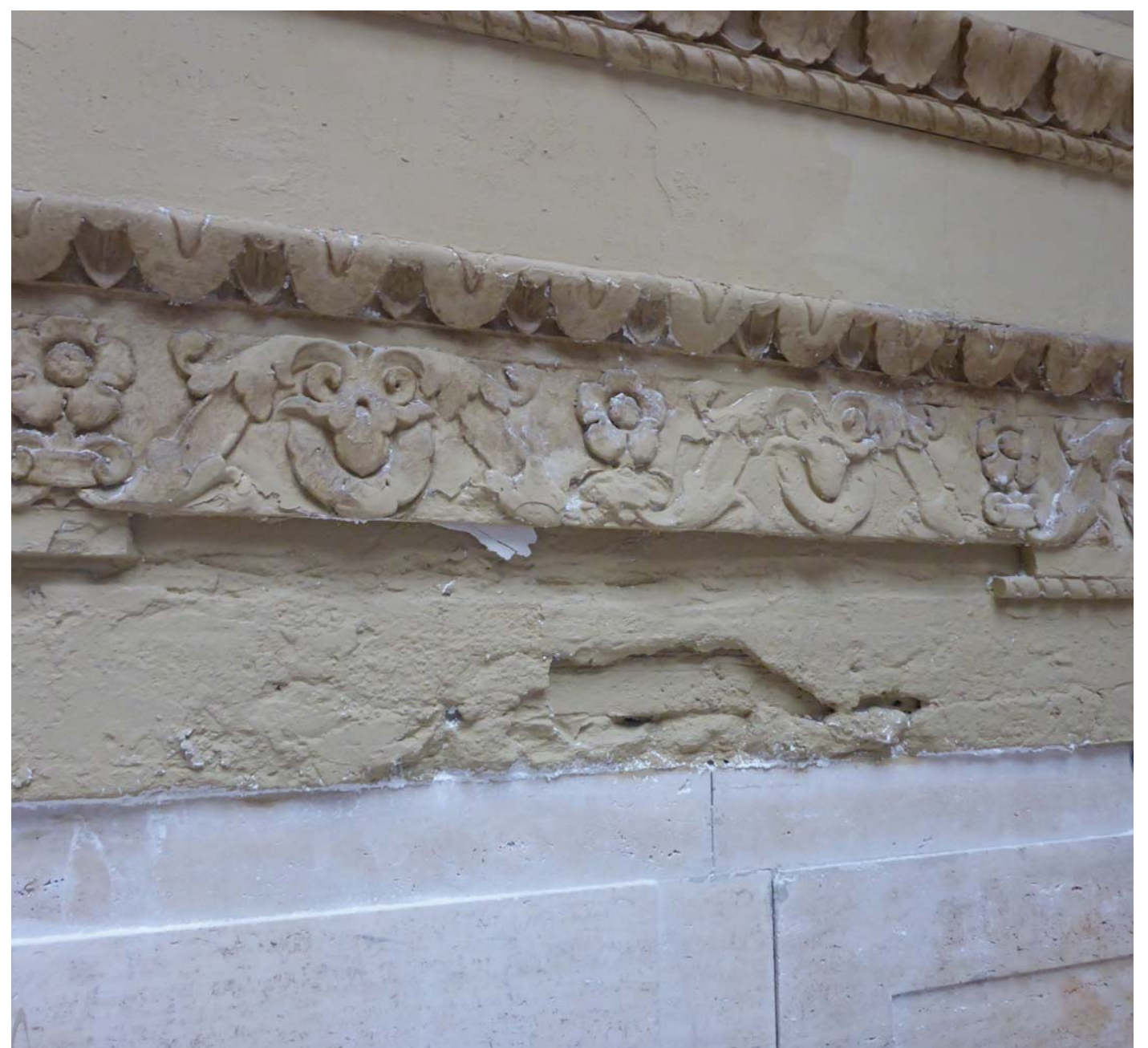
PLASTER DETERIORATION AT EAST WALL CORNICE
