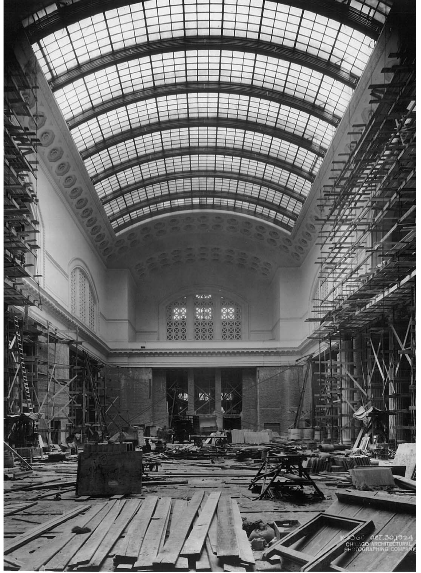
GREAT HALL CONSTRUCTION OCTOBER 30, 1924
