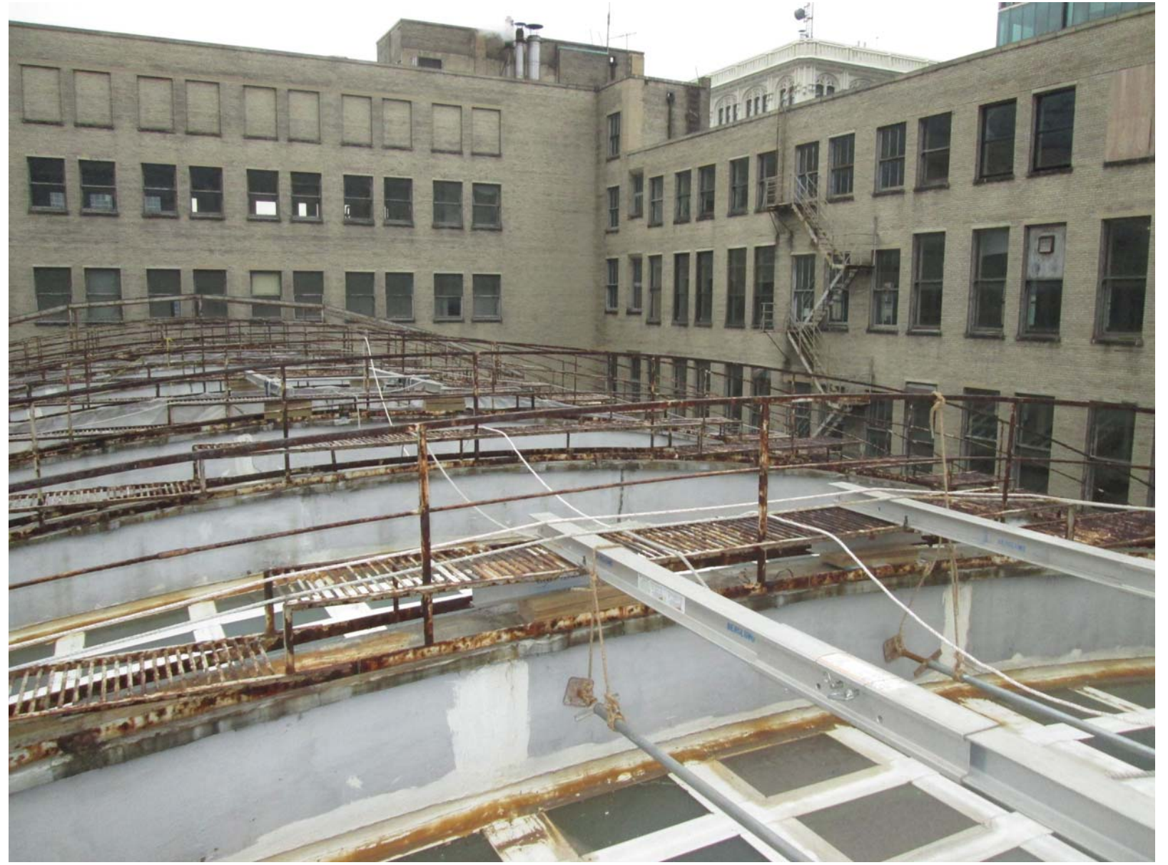
LIGHT COURT LOOKING SOUTHWEST OVER SKYLIGHT
