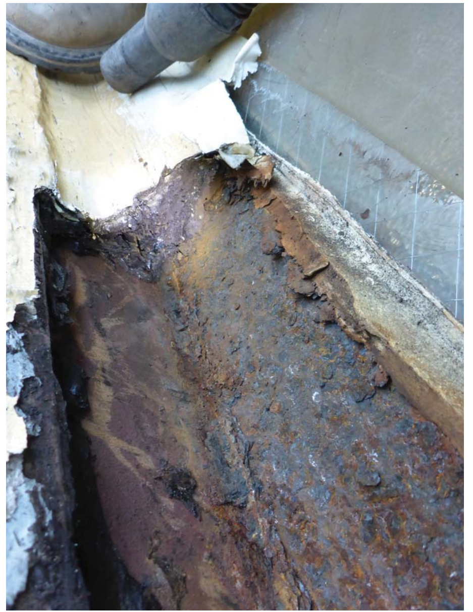
SATURATED EDGE FLASHINGS BETWEEN GIRDER AND SKYLIGHT GLASS
