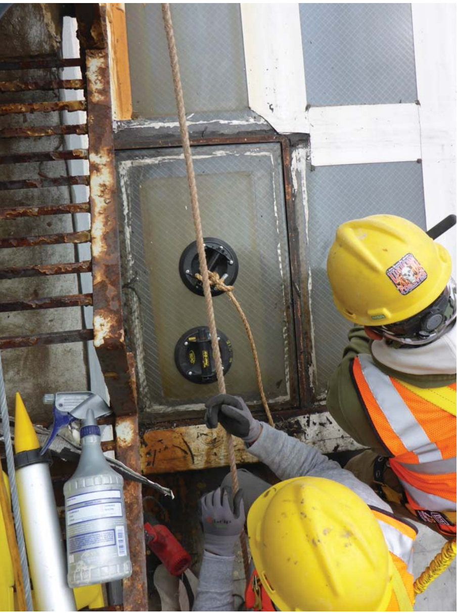
INITIAL GLASS REMOVAL
