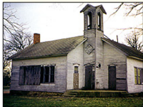
Chana Schoolhouse, Ogle County 1998 Endangered Building Grant Recipient
