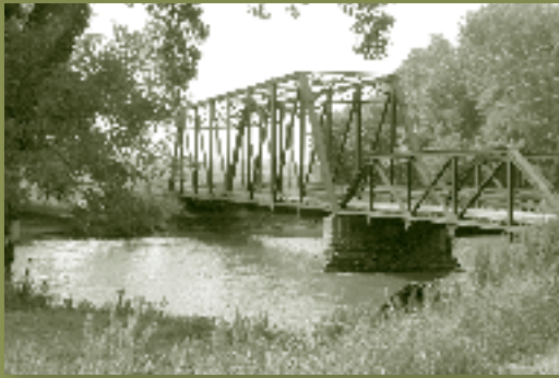
Spoon River Bridge, Bernadotte
